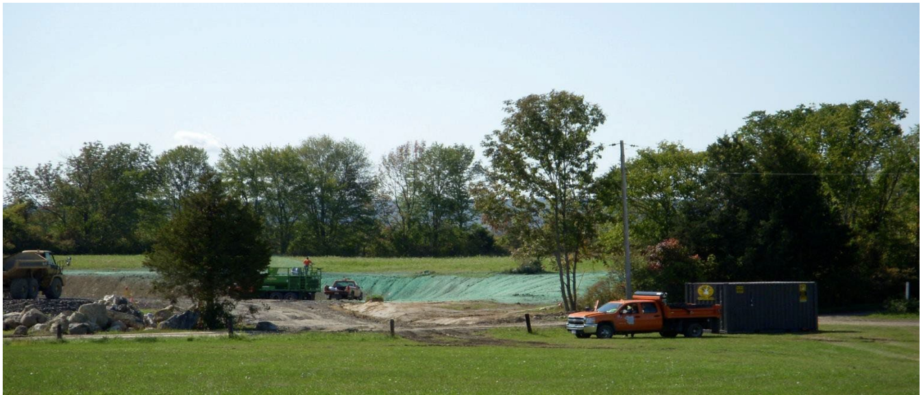
Hydroseeded Slope Stabilization
