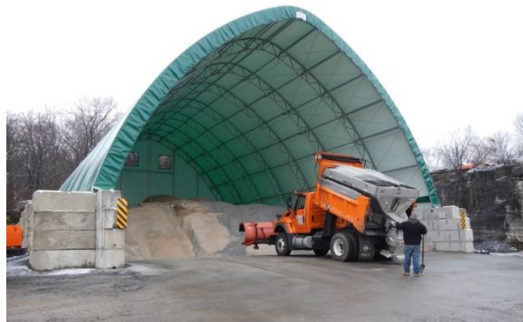
Salt Storage Shed
