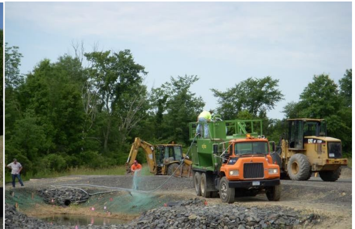
Hydroseeding Stormwater Pond Embankment
