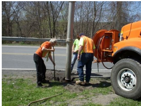
Catch Basin Cleaning
